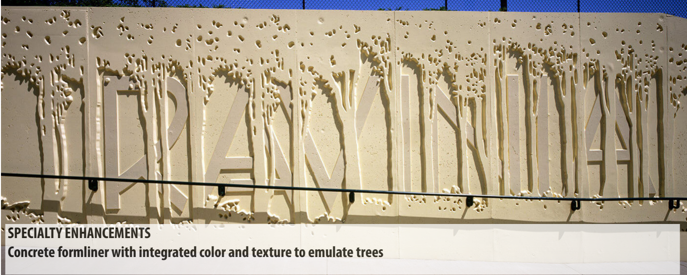
SPECIALTY ENHANCEMENTS Concrete formliner with integrated color and texture to emulate trees
